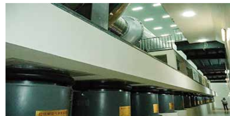
Ultra-large precision micro-vibration isolation platform based on air-magnetic hybrid array (40 m×7.5 m, floating weight 1,500 tons)
